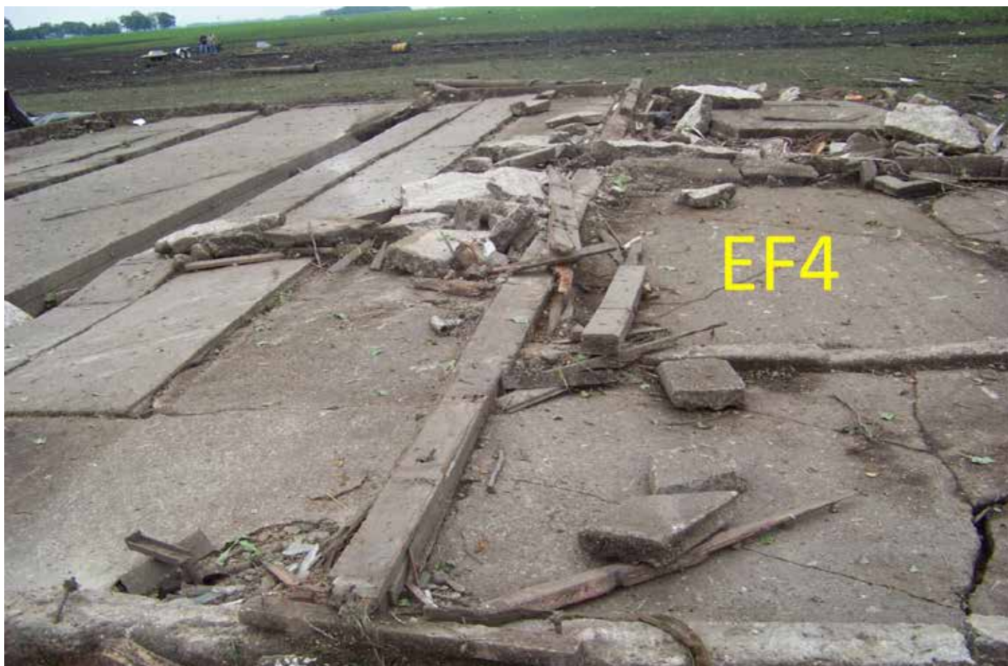
Figure 6.85k. A building completely sheared from its concrete slab from the EF3-EF4 tornado that struck North Dakota and Minnesota in 2010 (Source/Credit: NOAA).
