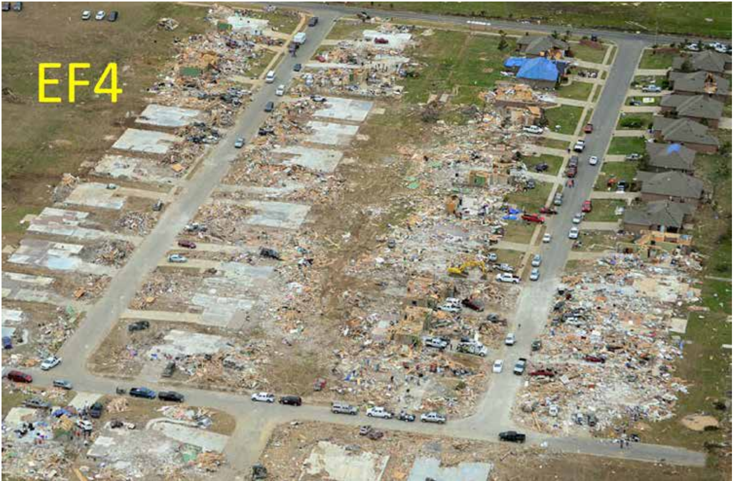
Figure 6.85l. A low, oblique aerial view of complete destruction of the Plantation subdivision near Mayflower, Arkansas from an EF4 tornado that struck on April 27, 2014. Most of the homes were leveled and swept clean off their foundations. Later inspection revealed a lack of properly constructed walls and foundation anchor bolts (Source/Credit: NOAA).
