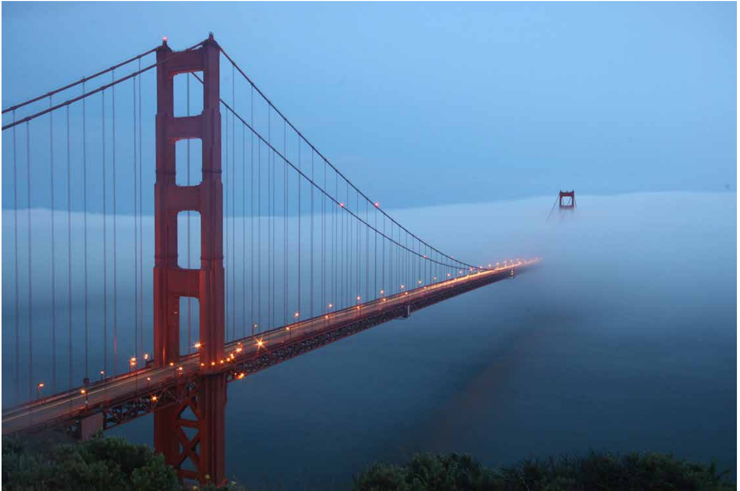
Figure 5.36. Advection fog that has developed in the marine layer. The fog in the distance almost hides one of the towers, which are 750 feet (230 m) above the ocean level. The top of the inversion is likely at about 750 feet. The image was taken on May 3, 2009. The Golden Gate marks one of the few gaps in the entire coast range system allowing the marine layer to occasionally penetrate inland to the Central Valley (Source/Credit: https://en.wikipedia.org/wiki/San_Francisco_fog#/media/File:Golden_Fog,_San_Francisco.jpg ).
