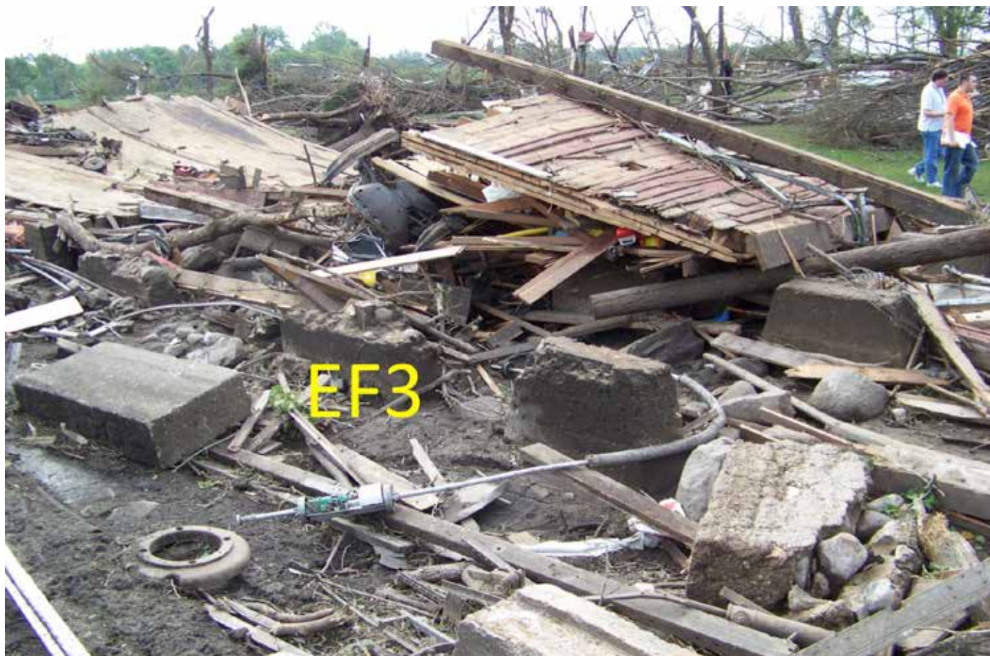
Figure 6.85i. Completely destroyed buildings due to an EF3 tornado that ravaged Wilkin, North Dakota in 2010 (Source/Credit: NOAA).
