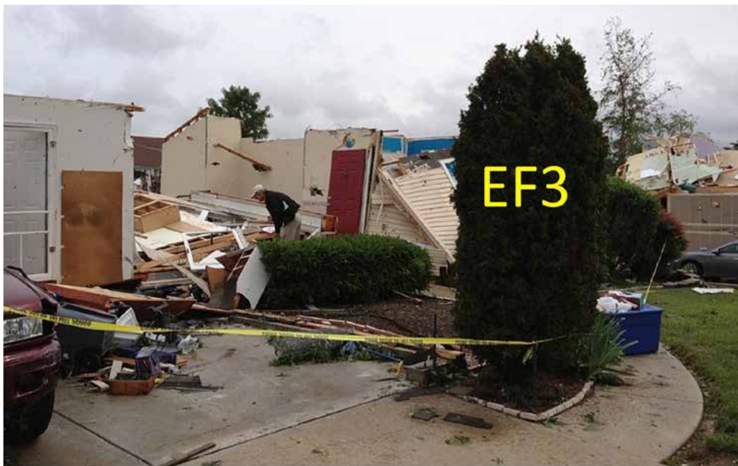
Figure 6.85h. An example of the kind of damage done by an EF3 tornado that hit St. Louis on May 31, 2013 (Source/Credit: NWS, St. Louis Missouri).
