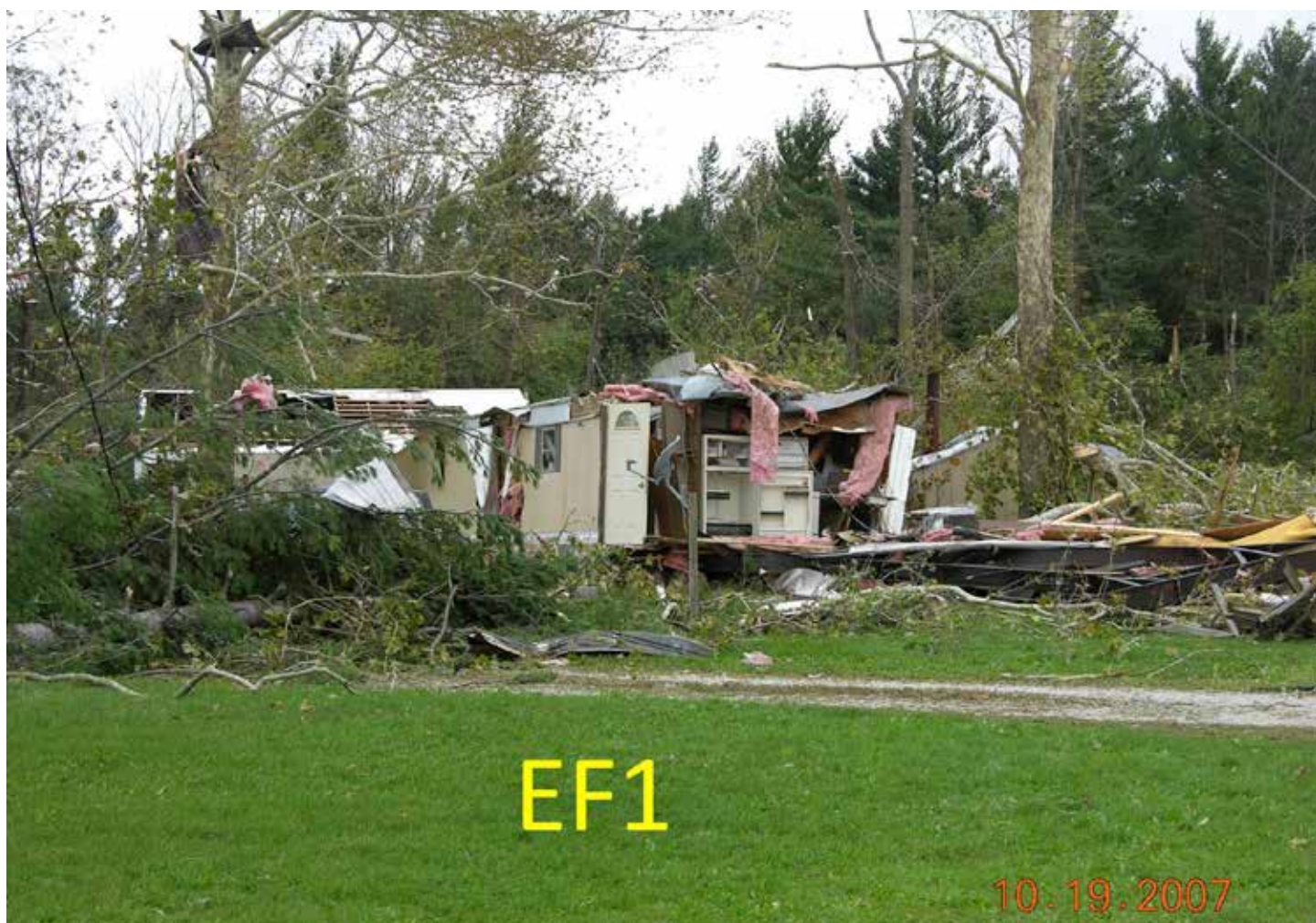
Figure 6.85d. Damage from an EF1 tornado in Indiana on October 18, 2007 included overturned single-wide and double-wide trailers and partially sheared trees (Source/Credit: NOAA).
