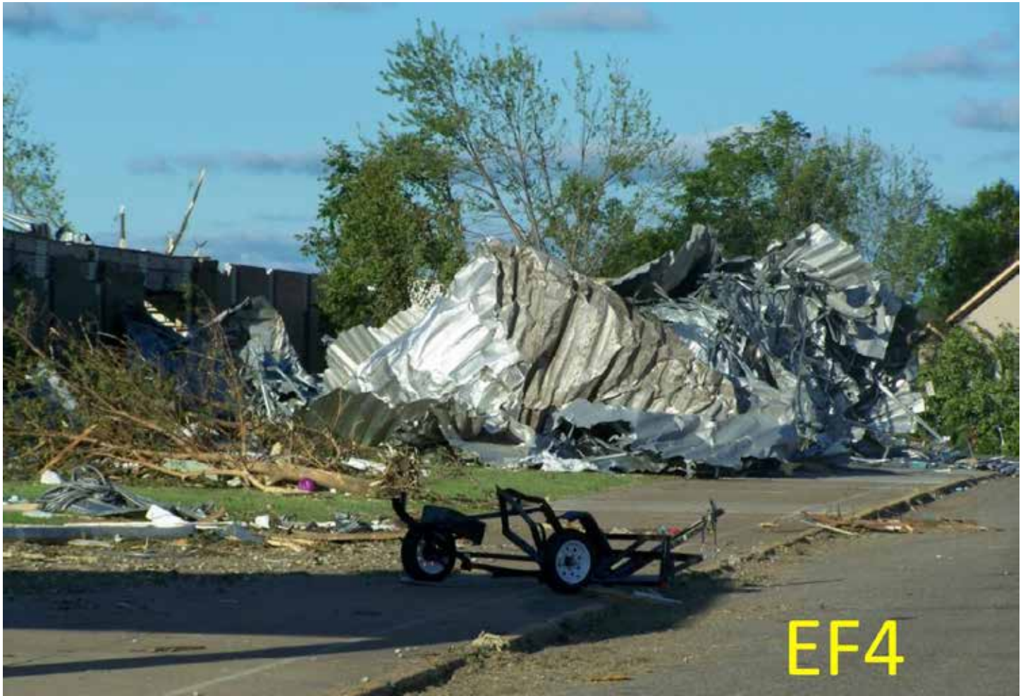
Figure 6.85n. Severe damage from the EF4 Wadena Tornado that struck Wadena County, Minnesota on June 17, 2010. The tornado had a maximum width of 1.1 miles/1.8 km and a track of about 10 miles/16 km (Source/Credit: NOAA).
